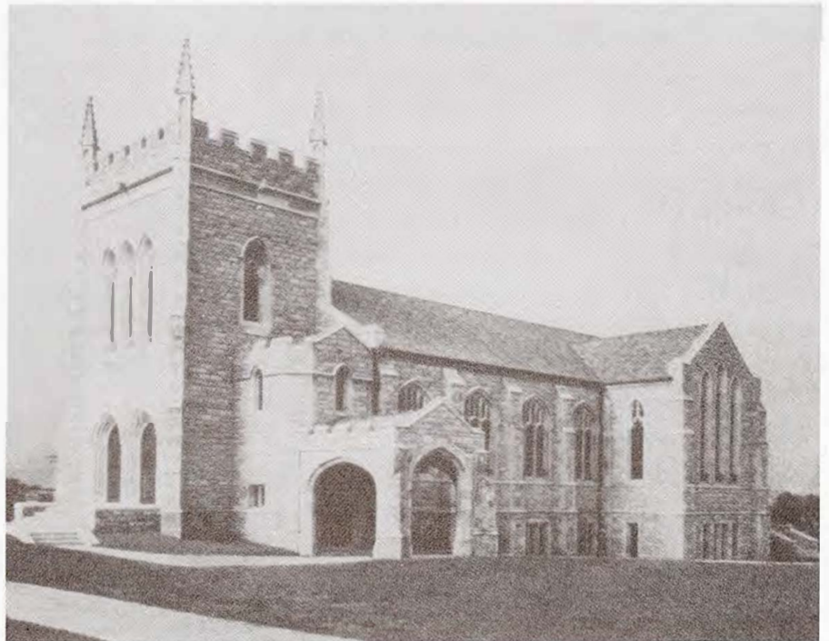
The newly built church called itself “The New Central Presbyterian Church of St. Louis” resulting from the merger between Central and the Clayton Presbyterian Church.
